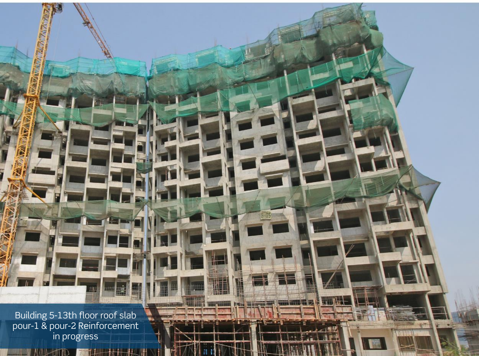
Building 4-13th floor Roof slab pour-1 & Pour-2 Reinforcement in progress
