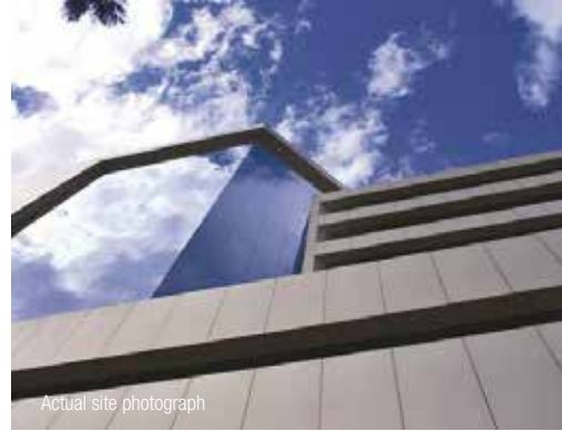
GODREJ CASTLEMAINE BUND GARDEN, PUNE
